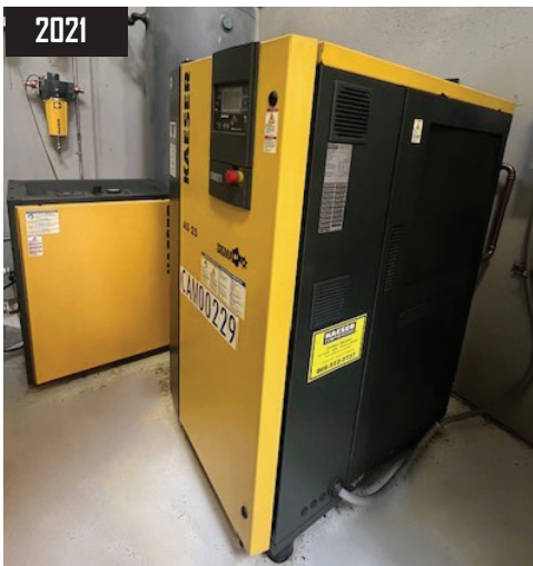
2021 Kaeser AS25 25Hp Rotary Air Compressor s/n 1491-7852940 w/ Sigma 2 Controls, 120 CFM @ 125 PSIG, 23.316 Run Hours, 9945 Load Hours, 2023 Kaeser Secotec TC36 Refrigerated Air Dryer s/n 1305-9040142, 240 Gallon Vertical Air Storage Tank.
