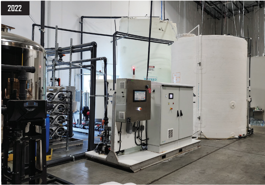
Omnilyte model Pro-4800 Alkalizer System with full RO System and Alkalizer, Dual Ozon System.
