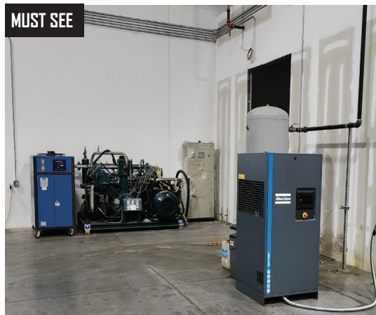
AF Oil Free Air Compressor for PET Bottling and Atlas Copco 50 HP Rotary Air Compressor.
