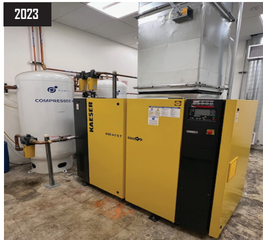
2023 Kaeser ASD 40ST SIGMA PROFILE 40 HP Rotary Air Compressor with Tanks
