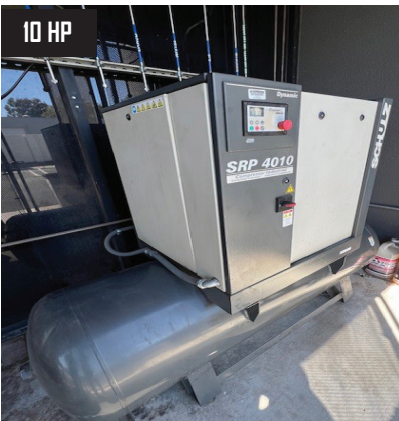
Schulz SRP 4010 10 HP Rotary Air Compressor and Tank.
