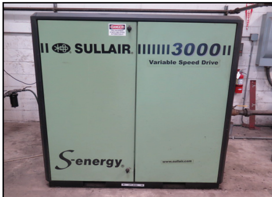
2018 Sullair 3000 II "S-energy" mdl. 3009V/A 25Hp Rotary Air Compressor w/ WS Digital Controls
