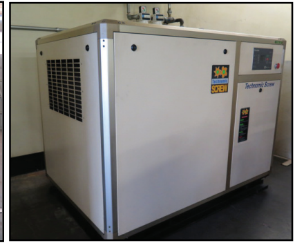
Coaire – Technomic Screw CHA-20S 20Hp Rotary Air Compressor
