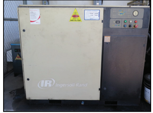
Ingersoll Rand UP6-50PR-125 50Hp Rotary Air Compressor
