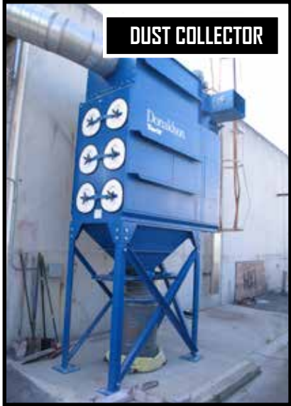
DONALDSON TORIT DOWNFLO-EVOLUTION DUST COLLECTOR MODEL DFE3-12 20 HP,
