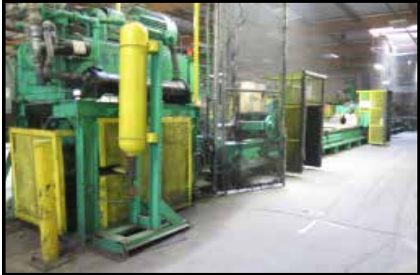
100 Ton Hydraulic Stretcher w/ Allen Bradley PanelView 600 PLC Controls
