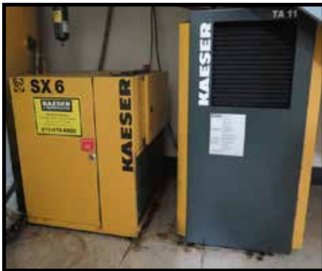
2001 Kaeser SX6 5Hp Rotary Air Compressor w/ Kaeser TA11 Refrigerated Air Dryer, 80 Gallon Tank
